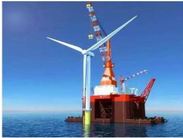
Figure 1. Wind power platform.
