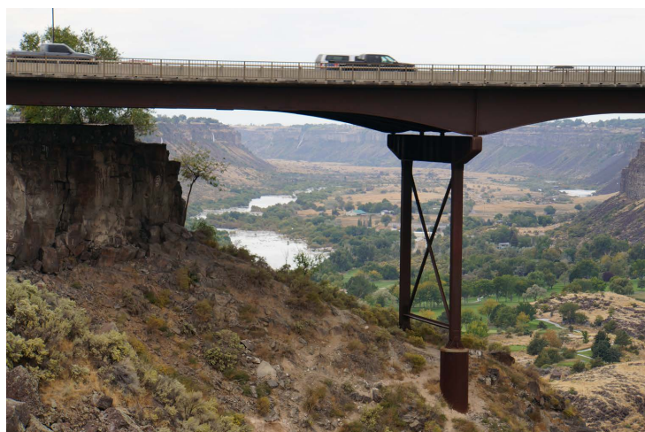
Figure 28. A highway bridge extending from rim to rim across the Snake River Canyon and the Snake River. Photograph by Lois Wright Morton.
