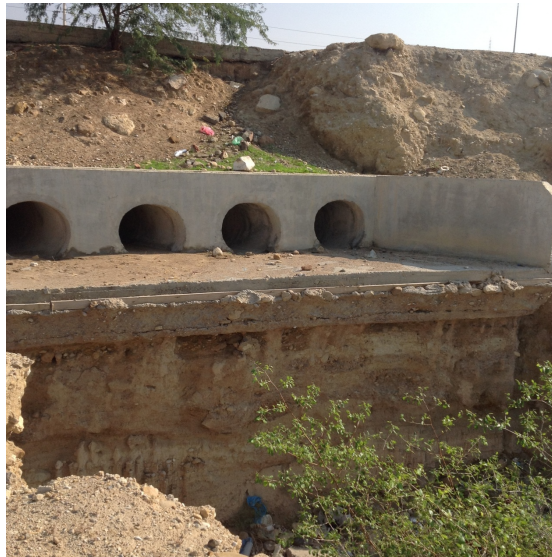
Figure 5. Head ward erosion in the immediate surroundings of the Dead Sea shore caused by the retreat of the Dead Sea (at around 500 m east of its present shore).
