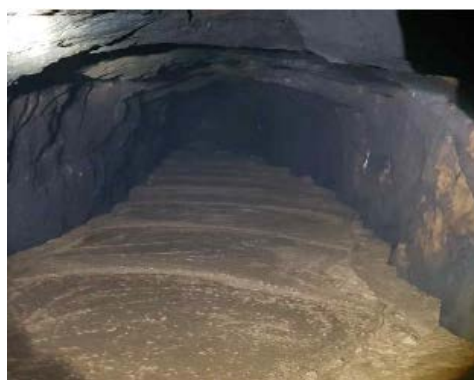
Figure 13. Formed concrete pouring.
