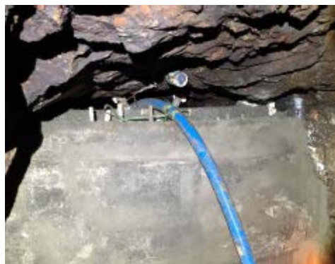
Figure 12. Introduction of formed concrete.
