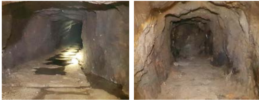
Figure 10. Tunnel in the mines.
