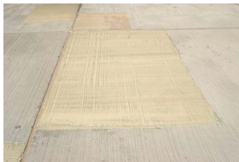
Figure 4. Conceret patche repaired (large size).
