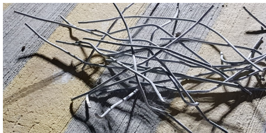
Figure 19. Reinforcement bars removed from pavement.
