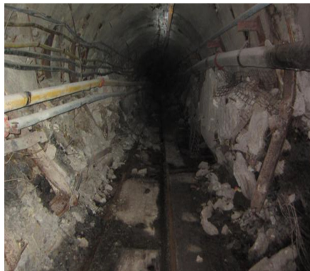
(d) The shed legs are twisted and squeezed in the spray layer falls off
