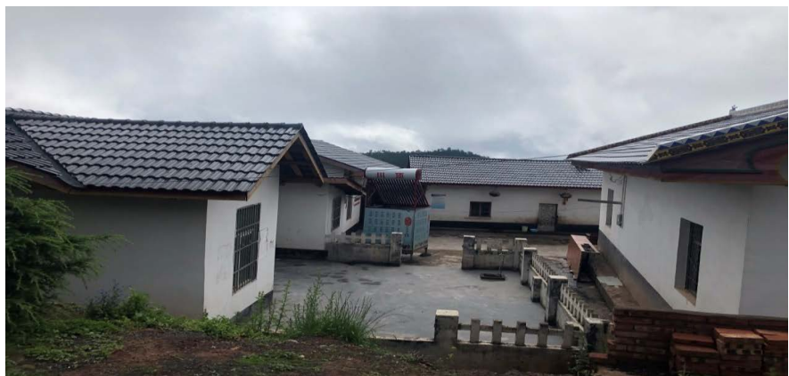
Figure 2. The buildings are directly painted with white paint (photo source: author self-photo).
