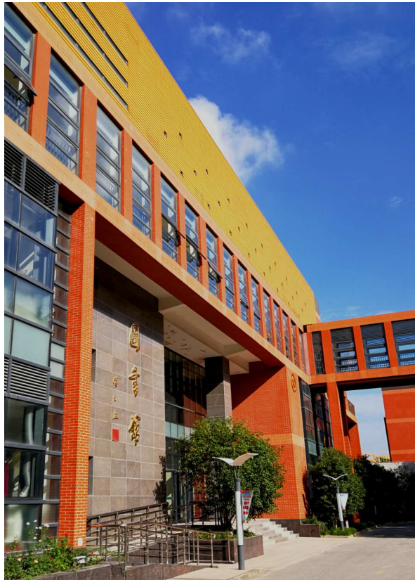
Picture 1. Xuhui campus library.
