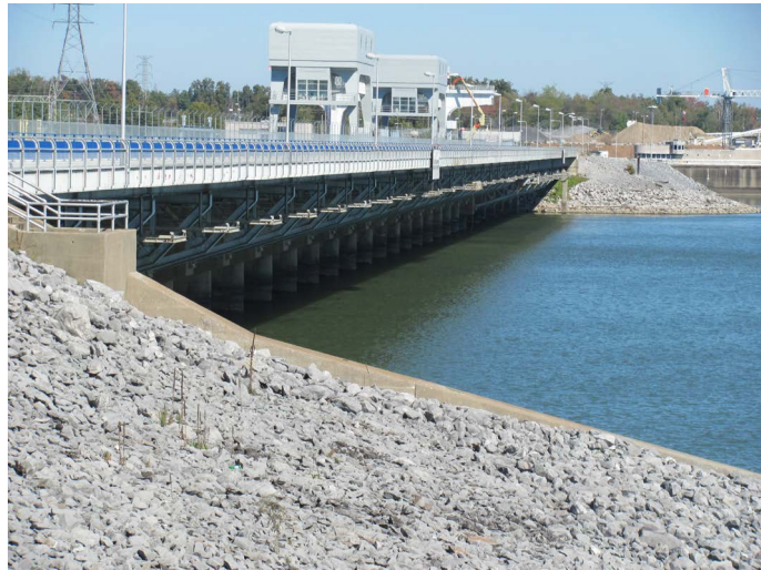
Figure 12. The Kentucky Dam at Gilbertsville, Kentucky was built on the Tennessee River 35 km upstream from its confluence with the Ohio River.
