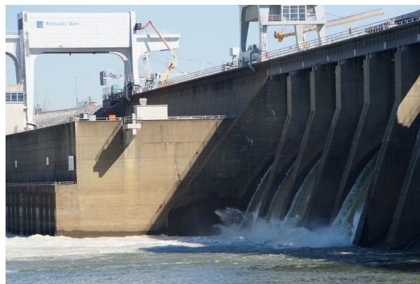
Figure 15. Kentucky Dam at Gilbertville, Kentucky was built on Tennessee River at mile marker 22. Photograph by Lois Wright Morton.
