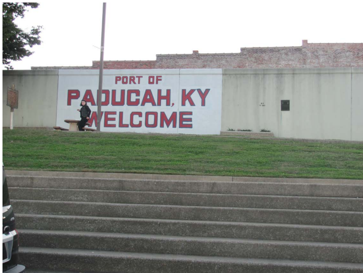
Figure 6. The river side of the floodwall at Paducah City Front during minor flood stage.
