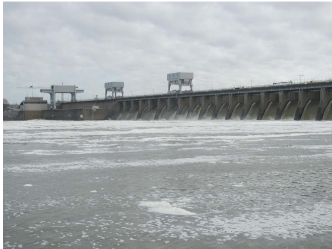
Figure 21. Kentucky Dam wide with gates open to reduce the flood pool on the Tennessee River after a major flood on the Ohio River.
