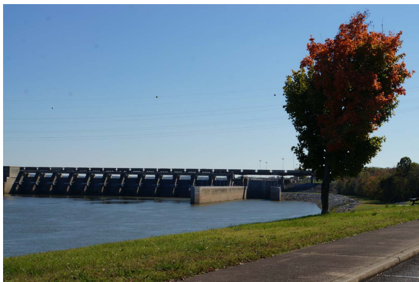
Figure 34. The railroad built above the Barkley Lock and Dam on the Cumberland River Barkley Dam and train. Photograph by Lois Wright Morton.
