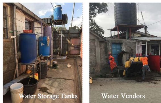
Figure 3. Water storage tanks and water vendors as sources of water.
