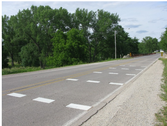
Figure 2. Transverse bars at community entrance.
