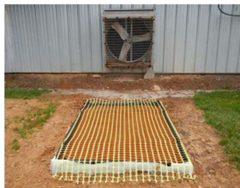
(c) Installed containment tray with red mud
