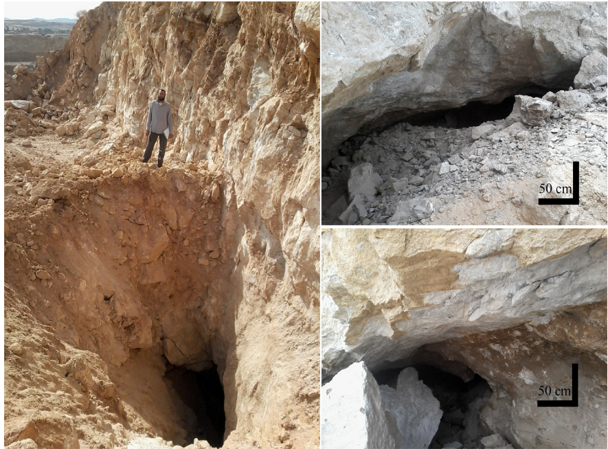
Figure 4. Field photos showing the presence of various underground cavities of different dimensions in the gypsum masses.
