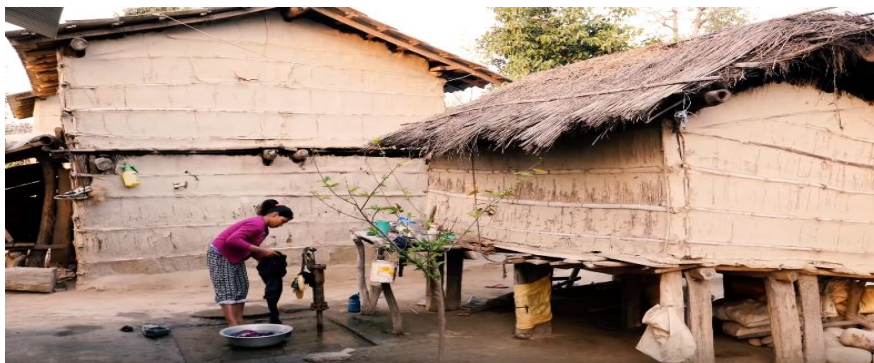
Figure 6. Two-storey house built by community peoples for emergency shelter (as a Preparedness measure).
