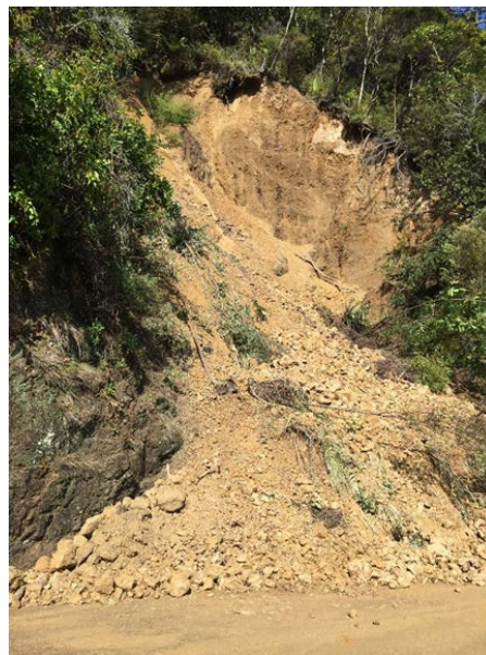
Figure 6. Over slip site 4.
