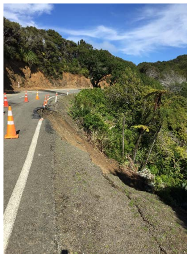
Figure 5. Under slip site 2.
