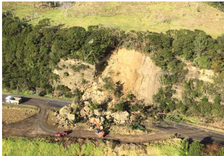
Figure 9. Site 8 rockfall (image courtesy of J. Griffith).
