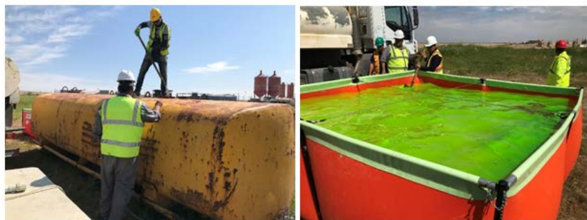
Figure 9. 18 - 24 dye test water tanks being prepared with green dye.
