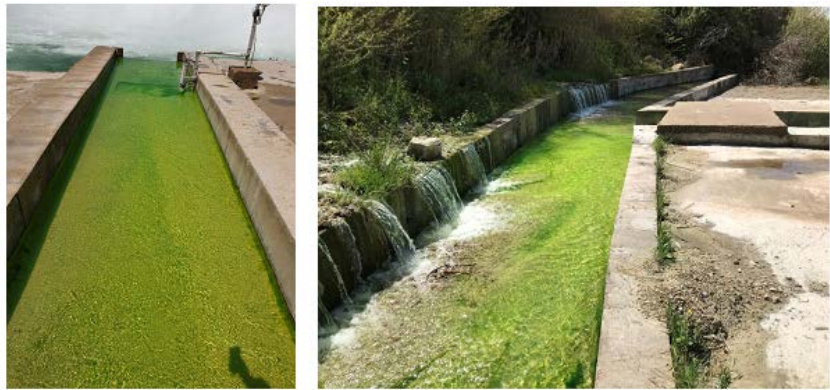
Figure 12. 18 - 24 dye test with green dye observed in Weir 4 on April 12, two days after injection.
