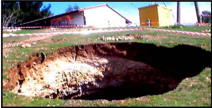
Figure 6. An example of sinkhole that appeared in 2003. The left bank sinkhole after full development.
