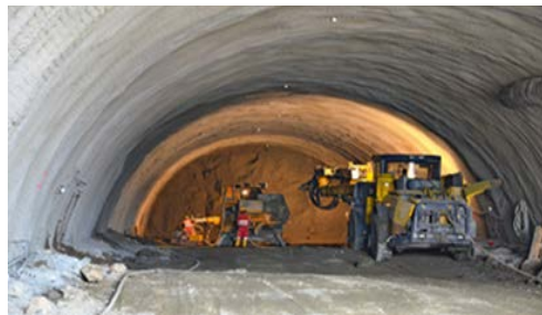
Figure 1. NATM (New Austrian Tunnel Method).
