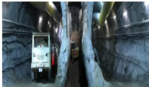
Figure 2. SEM (Sequential Excavation Method).
