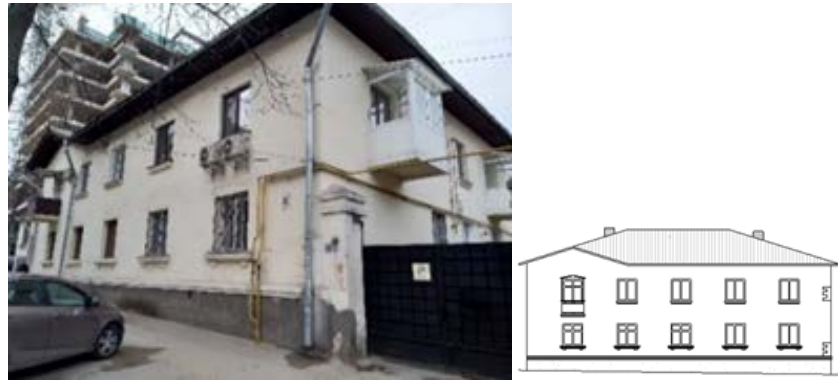
Figure 8. Architectural monument of local significance, 41 Vlaicu Pîrcălab Street (white and brown thetmopan windows; remodeled balconies). Source: original photo taken by the authors (March 2020), ( Monuments , 2011).
