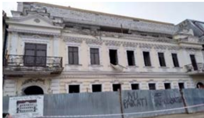
Figure 7. Reconstruction of the monument from Figure 6 with the addition of a level and attic. Source: original photo taken by the authors (March 2020).
