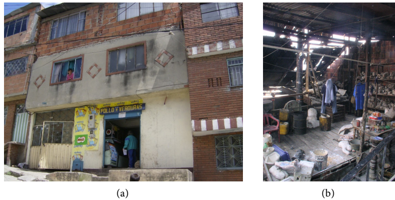
Photo 4. Typical rentals for commerce and production: In consolidated informal settlements, Bogotá. Left, (a): Three story home with rental general store (“Chicken and vegetables”); Right (b): Ceramics and Stucco “factory”/workshop [Author’s photos].
