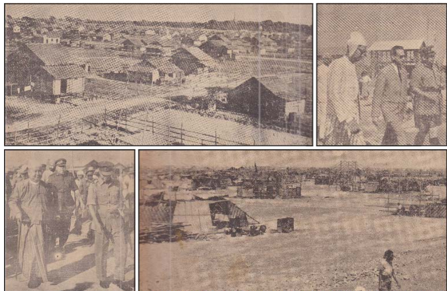
Figure 5. Historical Photos for Squatter Clearance in 1950s. Clockwise from Top-Left: 1) View on South-Okkalapa (1959); 2) Site Visit of UN Secretary General Desh Hammar-skjold; 3) View on Thaketa (1959); 4) Site Visit of Prime Minister U Nu. Source: (DUHD Library from Newspapers, 1959).
