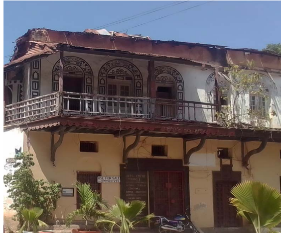
Figure 2. Building with detaching roof.
