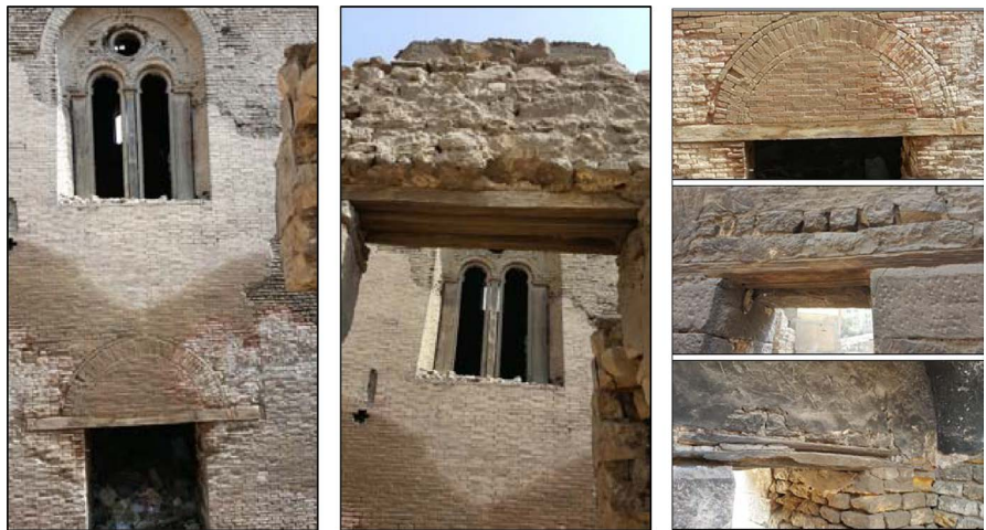
Figure 1. The wooden lintels at the mausoleum of Fatma Khatun.
