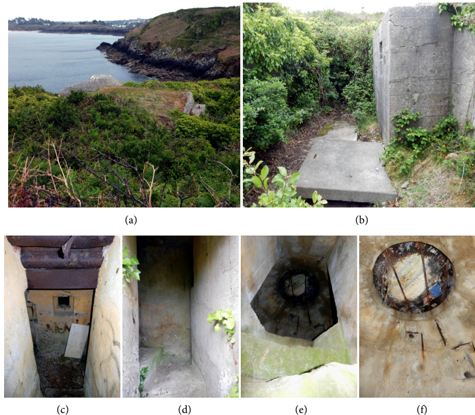
Figure 10. Eastern R601—(a) coverage and observation post, upper left Blanc Sablons; (b) PAK garage with covered access manhole to the ammunition room; (c) close combat embrasure; (d) access to the observation post; (e) observation post; (f) obstructed opening.
