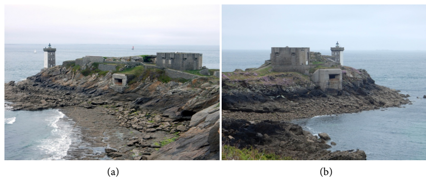
Figure 6. Fort de Kermorvan, Re112—(a) southern side view, 3 rd type, mod. 1846 crenellated guardhouse, southern bunker (65), lighthouse; (b) northern side view, crenellated guardhouse with leaning electric distribution cabin, northern bunker (64), lighthouse.
