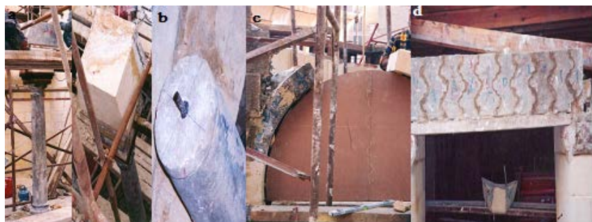
Figure 24. Reconstruction work of the façade.
