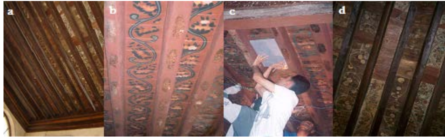
Figure 22. restoration work at the ceiling of Kutab.
