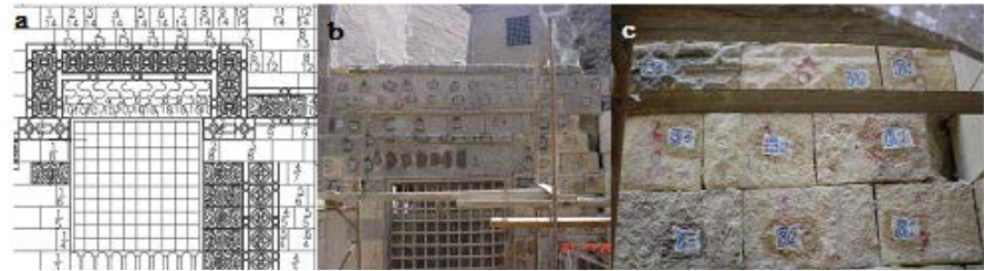
Figure 23. Numbering process for Façade elements on drawings and indicated in current position.
