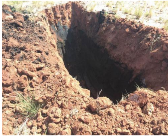
Figure 1. Sludge landfill upper layer covering soil 0.5 m.
