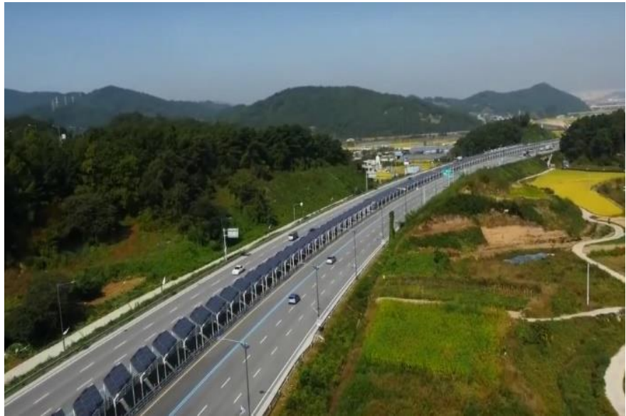
Figure 4. PV-covered bike lane connecting Sejong and Daejeon [20].
