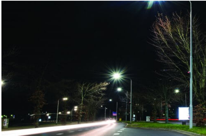
Figure 3. Twilight lighting controls in Nijmegen [19].
