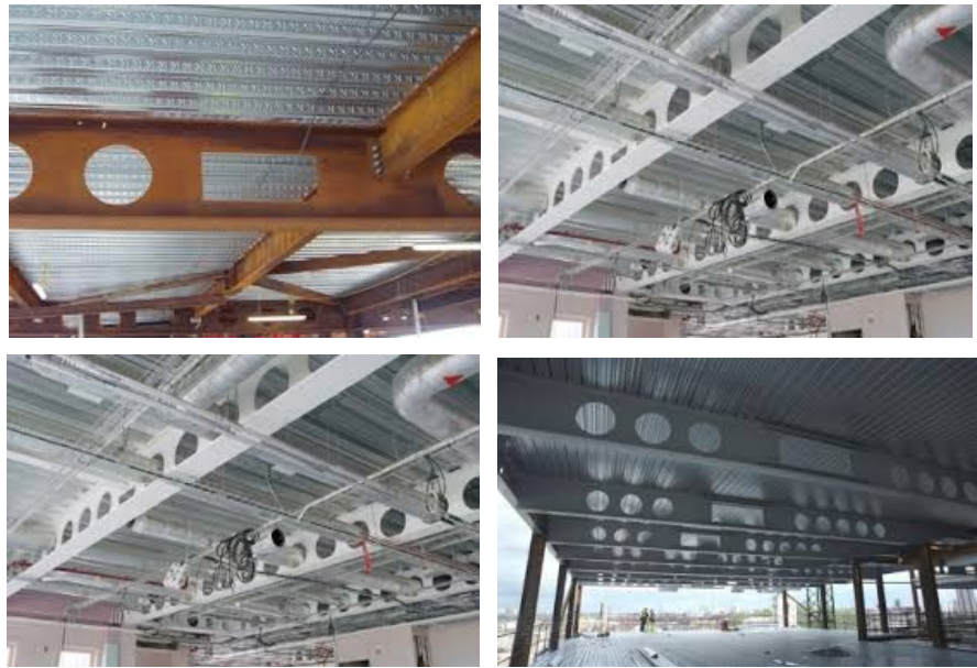
Figure 1. Web openings steel beam applications.
