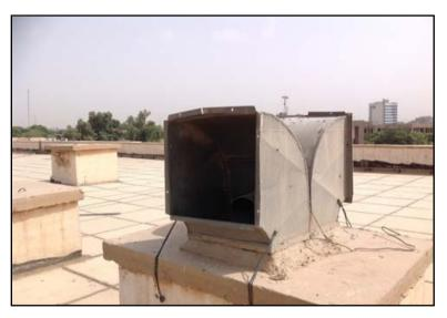
Figure 4. A duct which was not fitted with a barrier.
