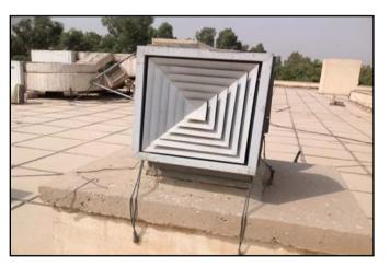
Figure 3. A discharge stack that had been fitted with a barrier.
