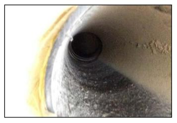
**Figure 1.** A white substance precipitated onto the internal surface of the ductwork.
