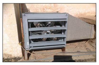
Figure 9. A set of fans have been installed at the end of the ducts.
