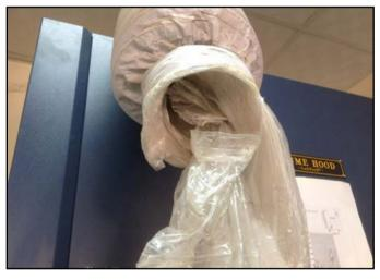
Figure 2. Plastic sheets were found inside the ducts.
