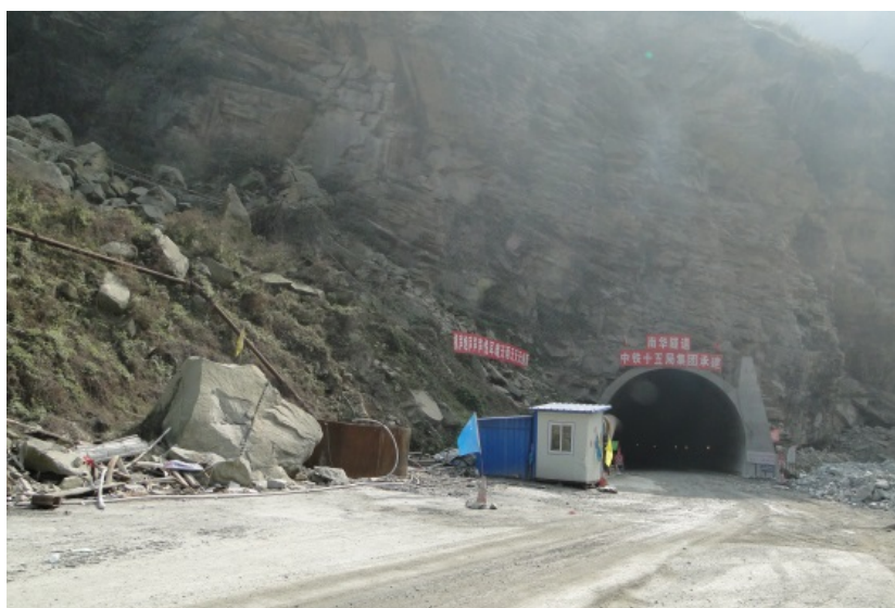
Figure 7. The portal of Nanhua tunnel before August 13, 2010.
