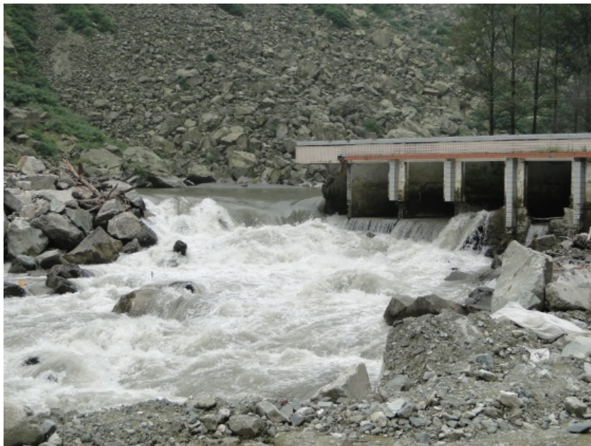
Figure 3. A quake lake formed by rock avalanche deposits submerged a hydropower station.
