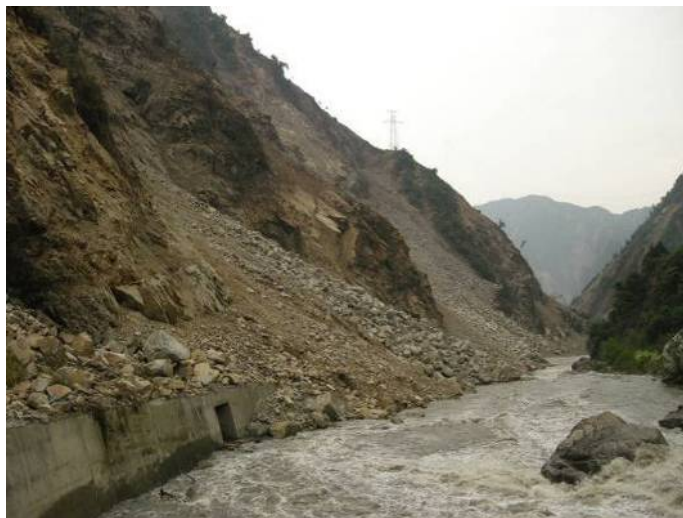
Figure 4. Rock avalanche buried the embankments.
