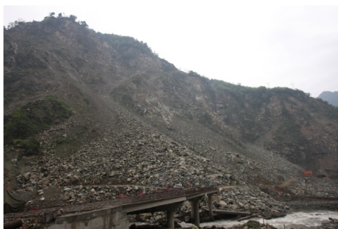
Figure 6. Rock avalanche fell from the steep slopes continuously, destroyed the bridge and buried a large section of road.
