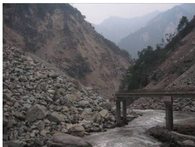
Figure 5. Rock avalanche destroyed the bridge.
