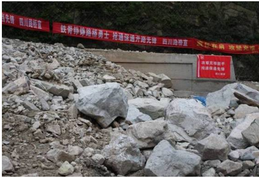
Figure 8. The portal of Nanhua tunnel was buried by debris flow deposits after August 13, 2010.
