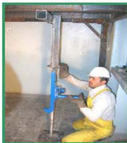
Figure 7. Lifting the roof of the structure by means of a jack.
