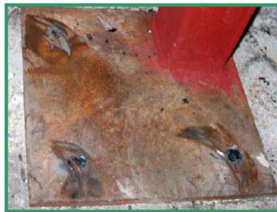
Figure 11. The upper surface of the column after finishing the work.
