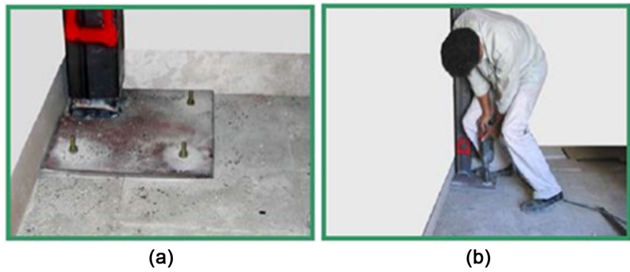
Figure 9. Piercing the floor mosaic and screwing the plate to the column.
