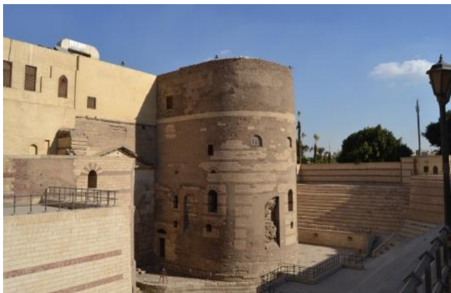
Figure 3. A roman towers underneath of the hanging church.
