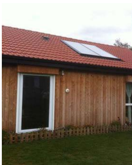
Figure 3. Solar wall on the House A.
