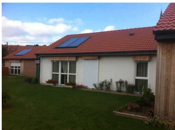
Figure 2. Solar wall on the House B.
