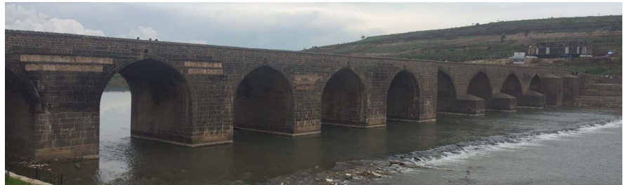
Figure 4. View of the downstream facade of the historic Tigris Bridge.
