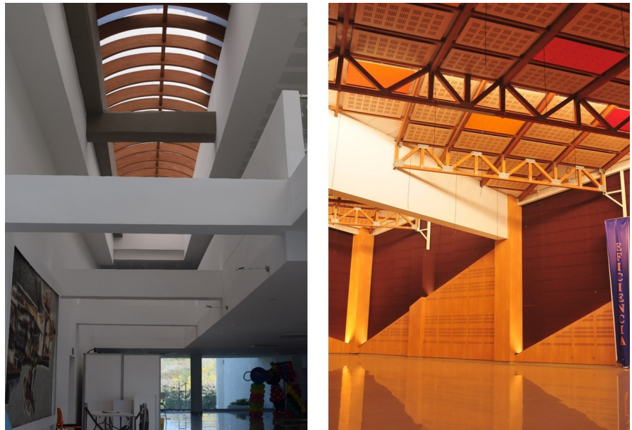
Figure 11. Cultural Center’s lobby and conventions room. Roof on reforested Wood structure designed to facilitate natural lighting of spaces, and in that way save energy costs. Source: Jose Carlos Gonzales Bell—Photographer.
