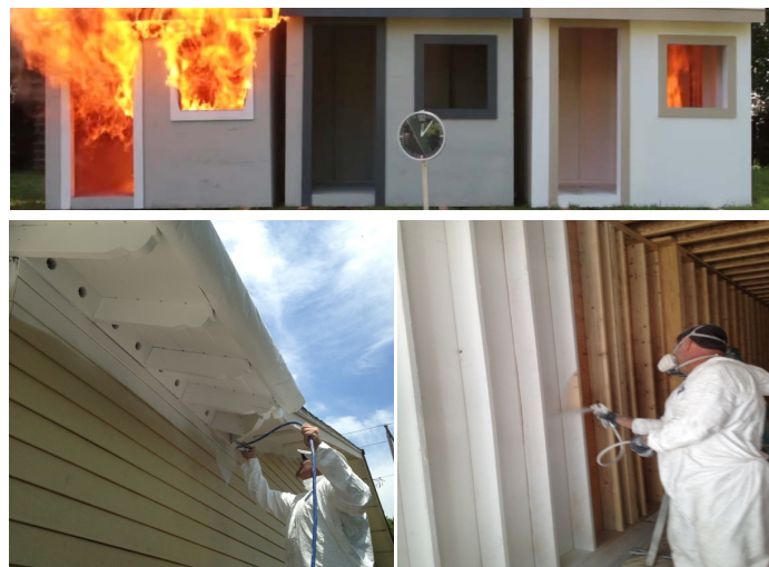
Figure 8. Performance of buildings with conventional and fireproof paints (Courtesy of Shield Industries, Inc. [24]).
