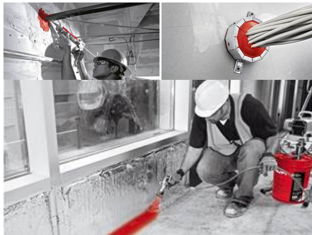
Figure 11. Application of firestops (Courtesy of Hilti https://www.us.hilti.com/content/hilti/W1/US/en/engineering/design-centers/firestop ).
