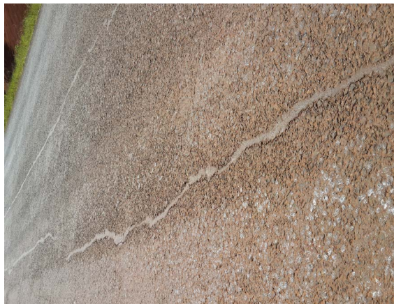
Figure 4. Sealed longitudinal cracks.
