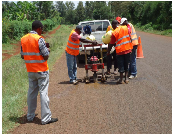
Figure 3. Core cutting on road surface.
