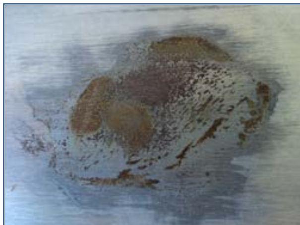
Figure 10. Aspects of galvanized steel sanding with formation of hydrated ferric oxide.
