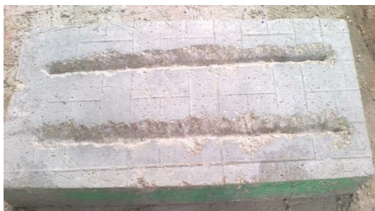
Figure 6. Drilled locations of steel rebars.
