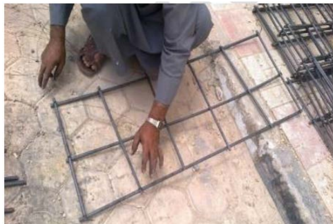
Figure 1. Slab reinforcement mesh.
