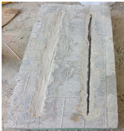
Figure 7. Embedding process of the steel rebars.
