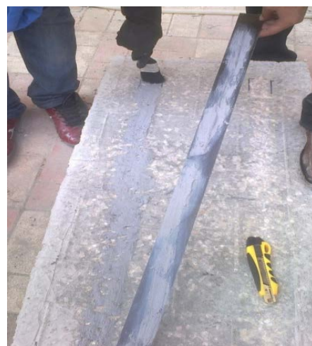
Figure 5. Installing of carbon laminate strips.
