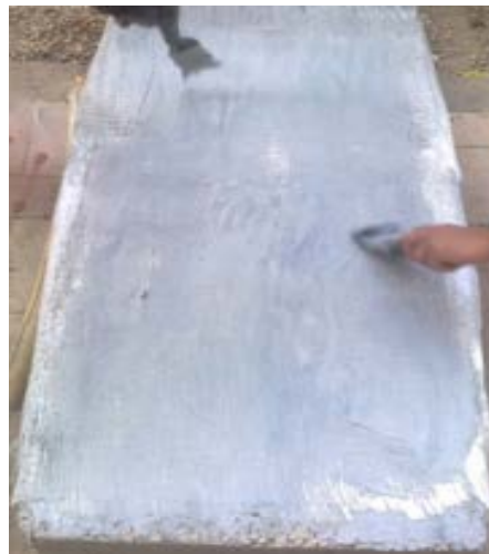
Figure 4. Installing of glass fiber sheets.
