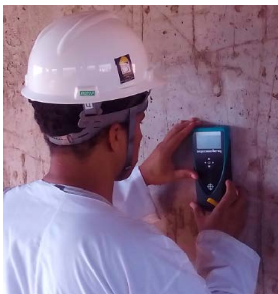
Figure 3. Electromagnetic detection test of the structural elements' rebar.
