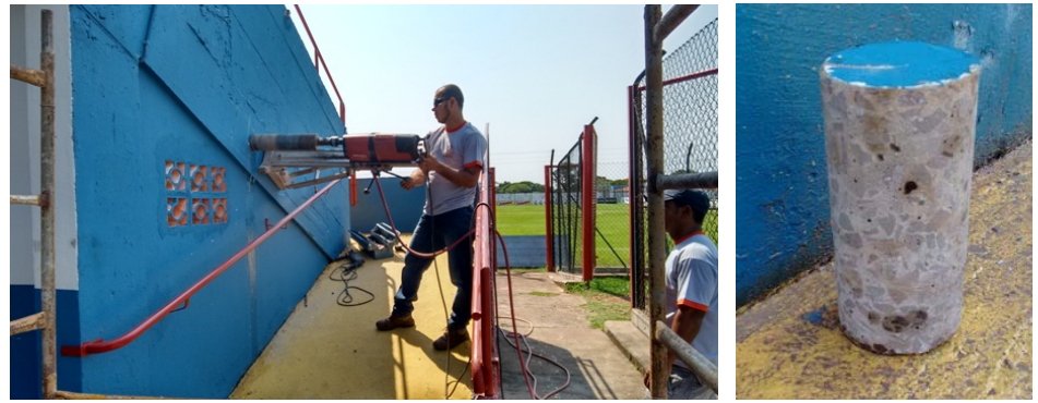
Figure 5. Extraction of specimens from the bleacher's structure.
