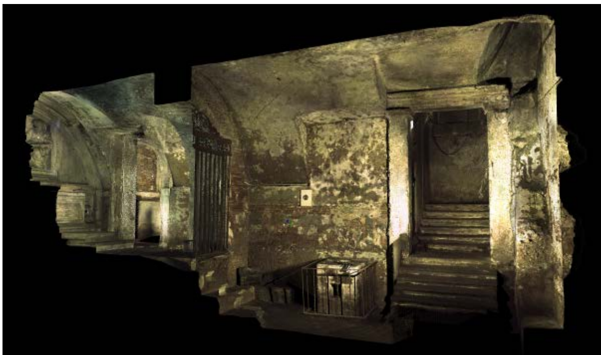
Figure 9. V and II compartment, the crypt of the Basilica of Santa Maria in Via Lata, Rome. Model three-dimensional perspective section.
