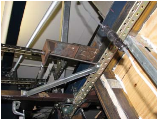
Figure 11. Attachment of threaded rod to the top spandrel beam of DRTF.
