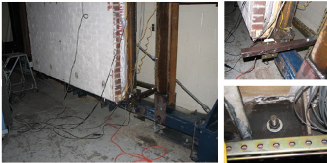
Figure 10. Attachment of the bottom channel to the lower spandrel beam of DRTF.
