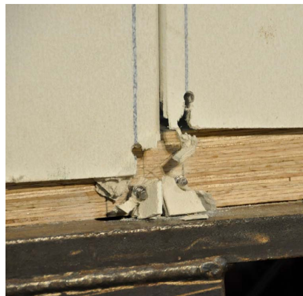
Figure 19. Tear off of CFB member from LVL frame.
