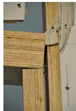
Figure 25. Apart of Panel-B from LVL frame opening (SWWOS). opening (SWWOS).
