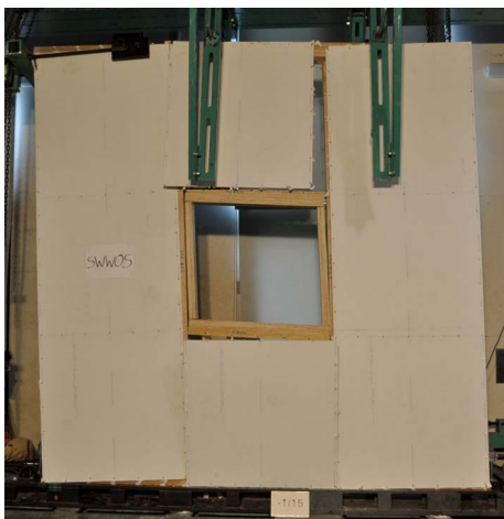
Figure 21. Final condition of shear wall with window type opening (SWWOS).
