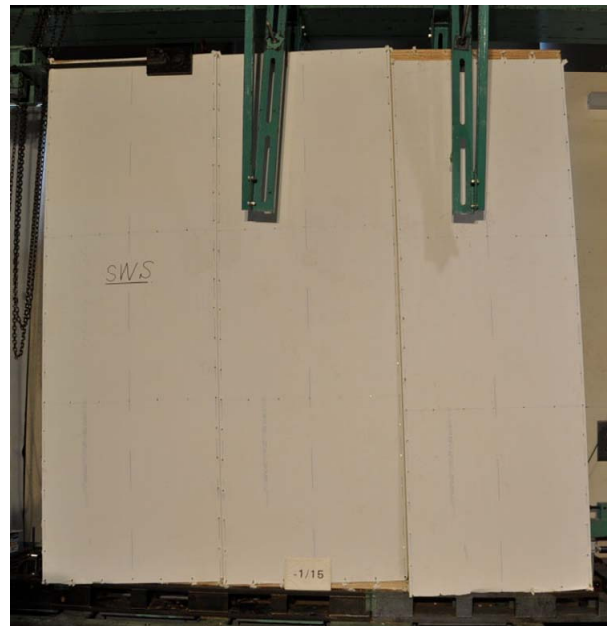
Figure 18. Final condition of shear wall type (SWS).
