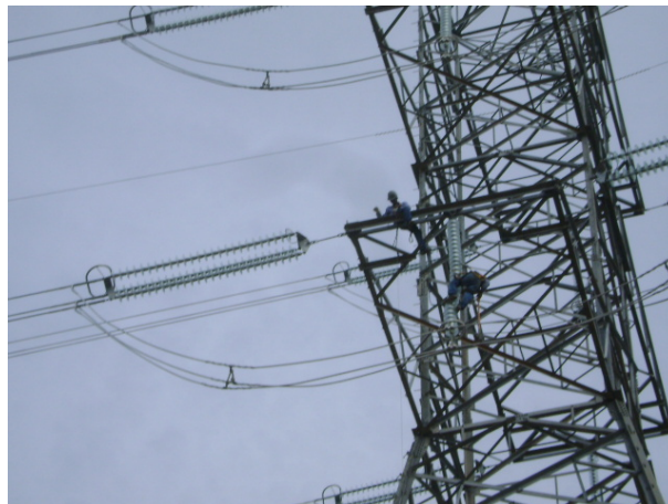
Figure 4. Connection of conducting cables to the measurement cable of the earth meter and preparation of conductors to measurements extraction.
