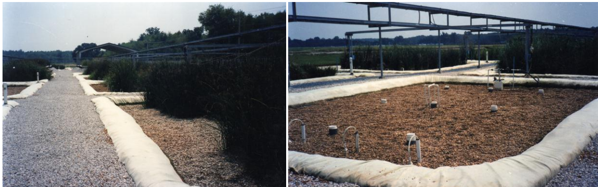
Figure 4. Engineered constructed wetland.
