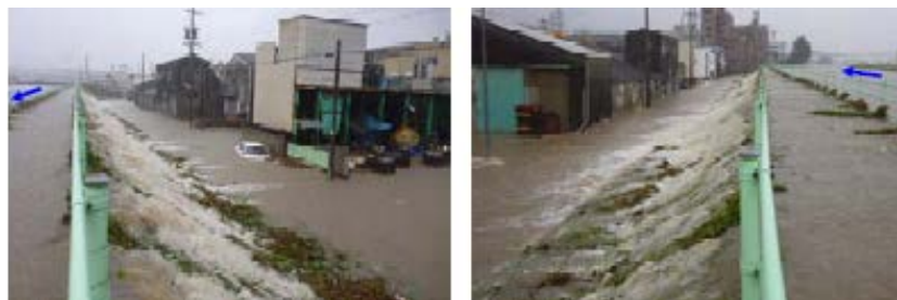
Figure 9. Overflowing from top of the levee in Hatta River.
