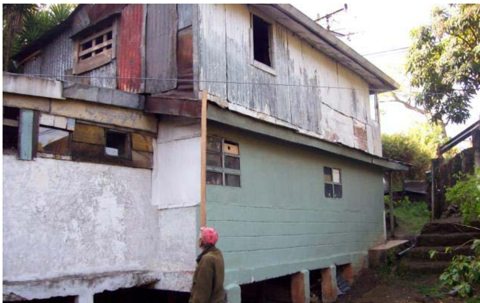
Figure 4. Flooded area in Rincón de Ricardo. Local resident Helio Fonseca shows the level reached by the water during the flood of July 2010.
