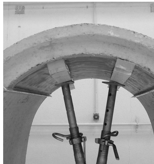
Figure 9. Placing the carbon plates.
