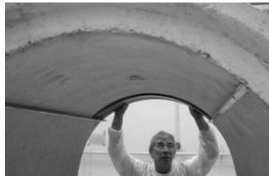
Figure 8. Fitting the brackets.
