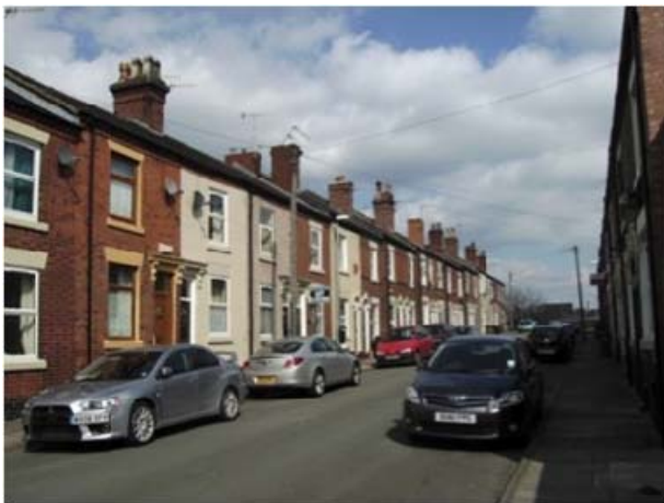
Figure 3. Small terraced houses in Stoke-on-Trent, UK.
