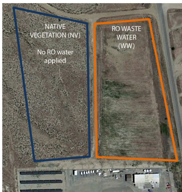
Figure 1. Aerial view of reverse osmosis (RO) plant and field (right) receiving the application of RO reject waste water (WW) and adjoining un-cultivated field of native vegetation (NV) used for comparative purposes.
