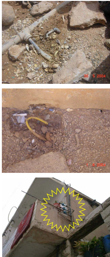
Figure 8. Examples of administrative loss in Mafraq: left-the meter is removed and replaced by a T-joint; middle-pipe connection passing the meter; right-connection to supply the housing unit before the meter.
